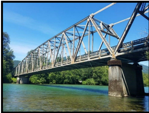
Marblemount Bridge – Skagit River
