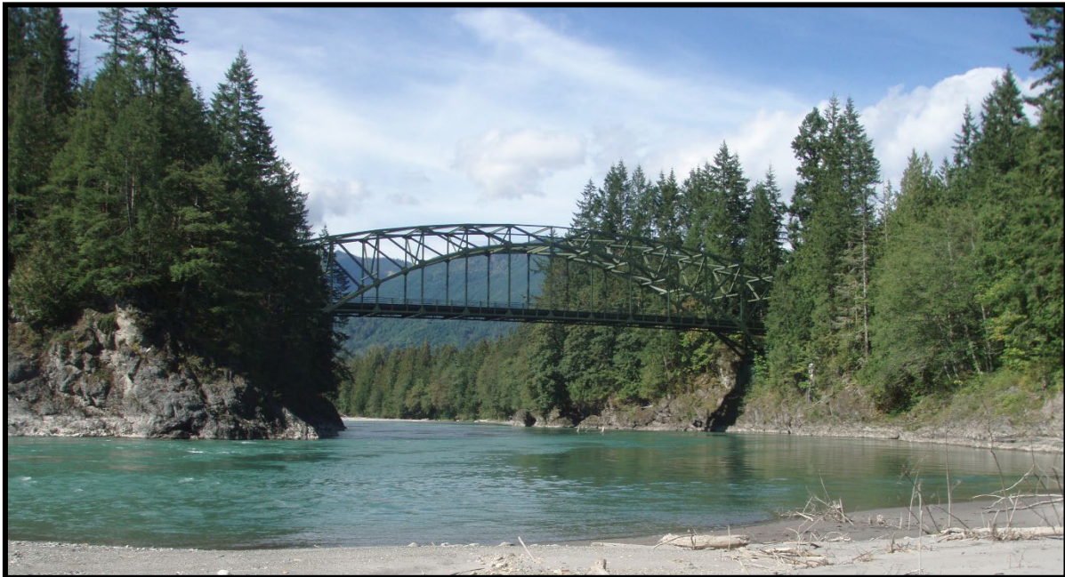
Dalles Bridge near Concrete (Concrete-Sauk Valley Road)
