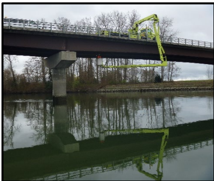
S Fork Bridge, UBIT inspection
