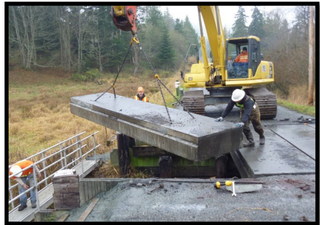
Campbell Lake Outlet receiving new timber cap, 2013
