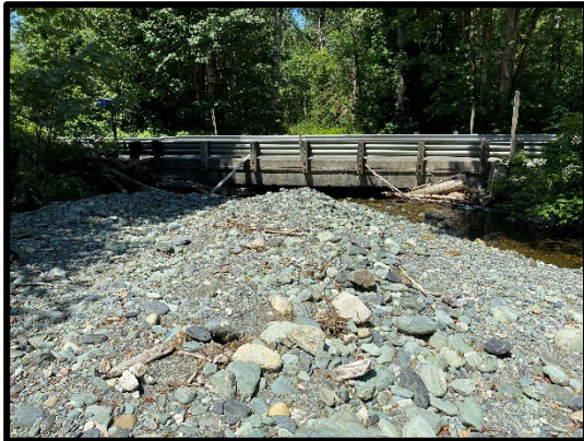
Mill Creek channel upstream of bridge.
