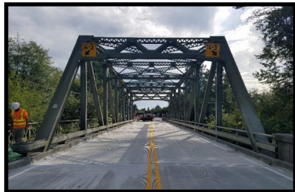
Samish River Bridge - Vertical Clearance Signage
