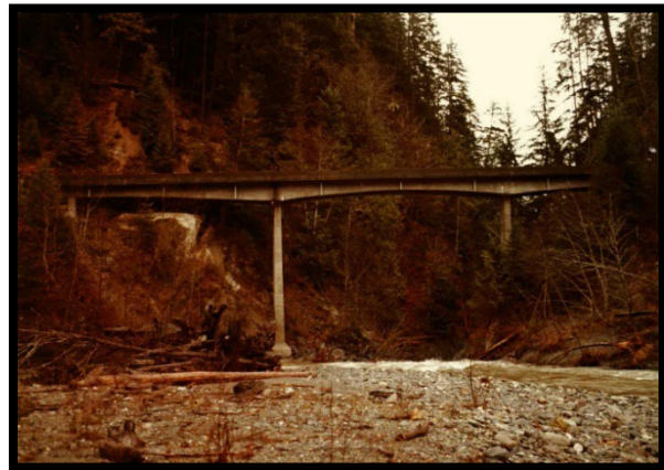
Upper Finney Creek Bridge
